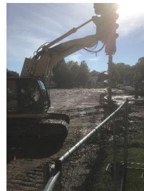
Installation of Geopiers
