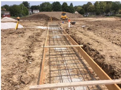
Formwork and rebar installation for gym addition
