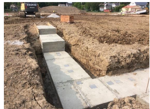
Footings for gym addition getting poured
