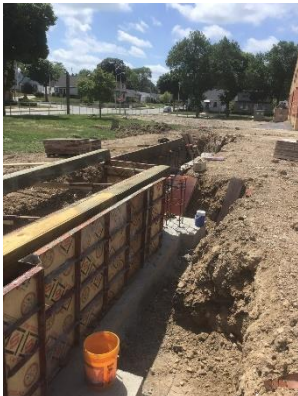
Formwork for frost walls on south end of Building B
