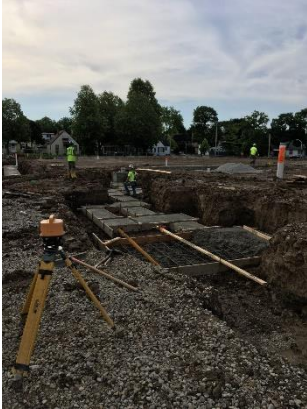
Footings being poured along North side of Building B
