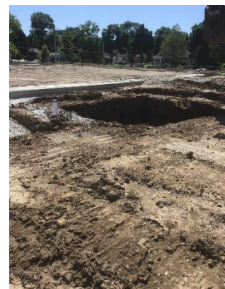
Excavation for Elevator pit
