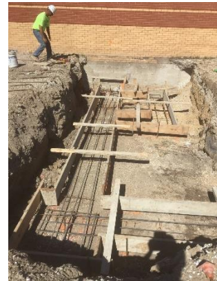
Formwork and rebar install where Building B meets Building A
