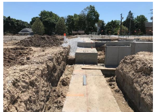
Angles for precast installed
