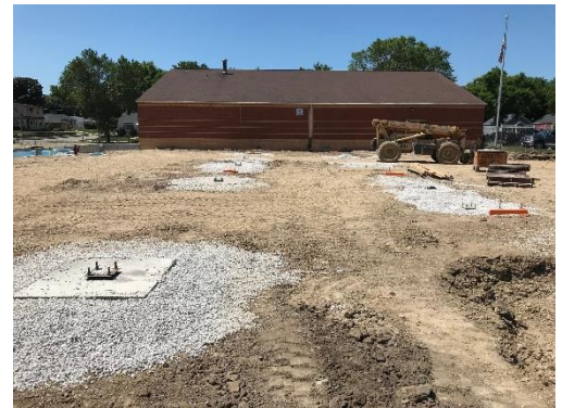
Column pads poured and base plates set
