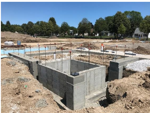
Elevator pit poured
