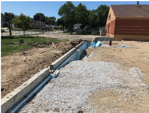
Installation of insulation and backfill
