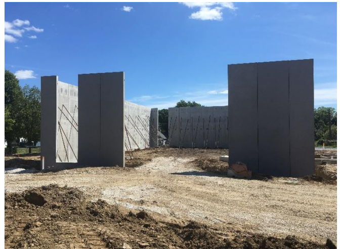
North face of gym
