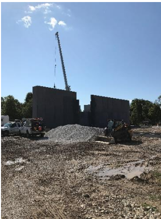
West face of gym
