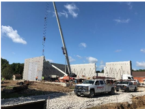
Northeast corner of gym
