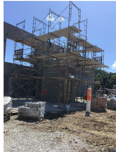
Elevator and stairwell
