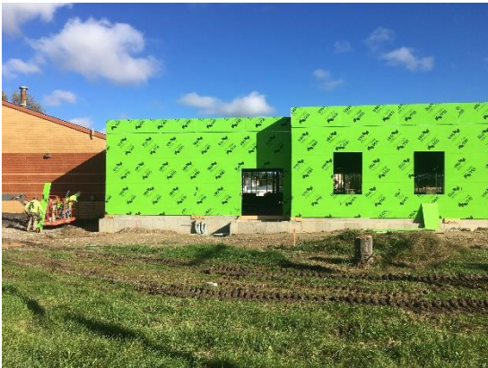
Dens glass sheathing being installed
