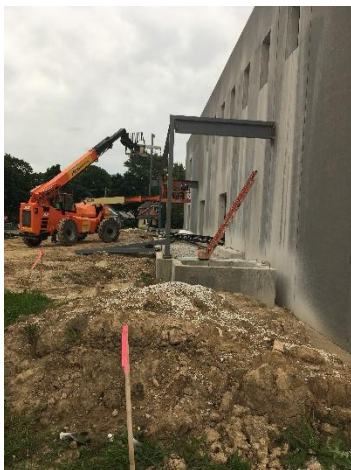
Steel for gym storage now set
