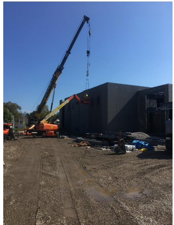
Last precast panels set on gym
