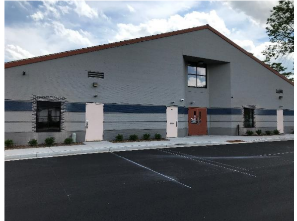
New windows installed in existing building
