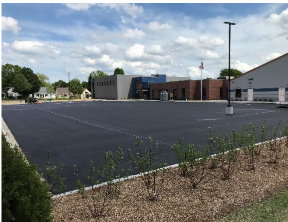
Finish coarse of asphalt is installed
